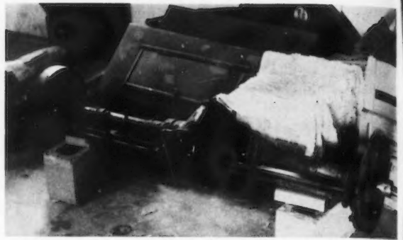
Substituted axle on 1912 Mitchell Getabout roadster identified as a Weston-Mott.
